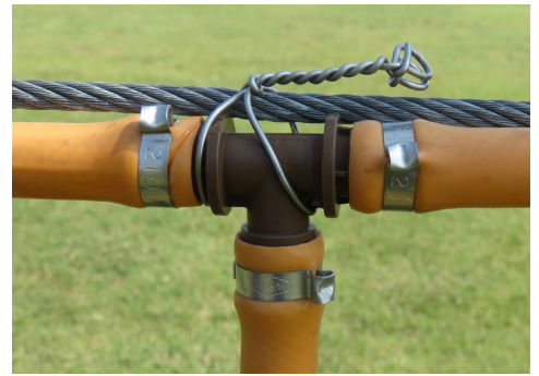
(Above) Place pinch clamps on each connection before inserting fittings, and secure all joints with wire ties.
