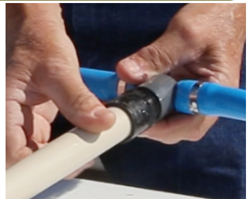
(Above) After manifold is attached to 1/4" lateral cable on pivot, screw in Dragon Drops.
