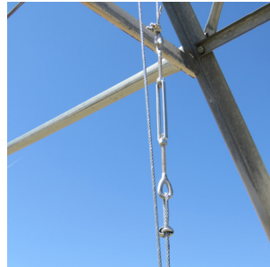
(Above) Close up of turnbuckle on tower termination.
