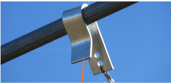
(Above) Using the Truss Rod Assembly Tool, slip truss rod clip onto truss rod and repeat on opposite side.
