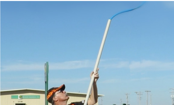
(Above) Slip PVC sleeve over drop hose.
