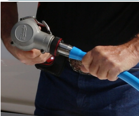
(Above) Use ProPEX tool to expand ends of drop hose and insert fittings.
