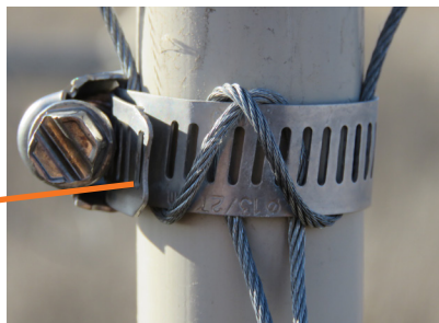
(Above) Take truss rod cable and slip folded point into 1 1/4" screw clamp. Insert cable back through clamp and tighten screw clamp with cable inserted.
