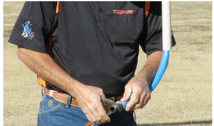
(Above) Insert 3/4" Adapter MPT x HB and secure with 3/4" pinch clamp.
