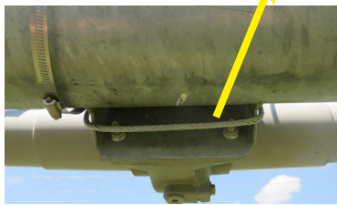
(Above) Close up of cable wrapping around motor bracket.
