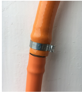
(Above) Place insert coupling into flex hose/emitter tubing, secure with 1/2" pinch clamp on flex hose side.
